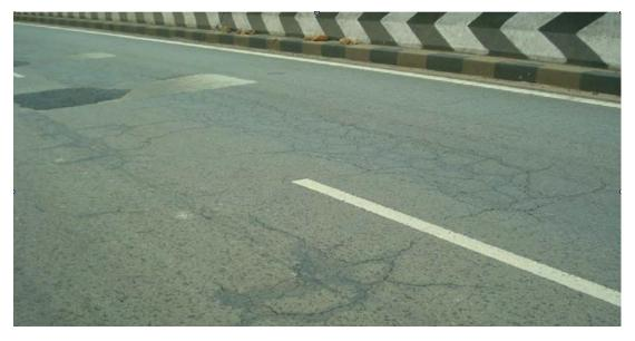
Fig. 1 rutting and cracking along wheel path at Km 53.00 Chennai-Tada road, N.H.5
