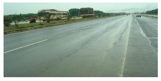
Fig. 4 Longitudinal cracks at Km 36 Chennai-Tada road, N.H.5
