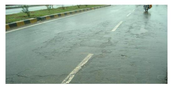
Fig. 3 Severe map and block cracking at Km 32.350 Chennai-Tada road, N.H.5
