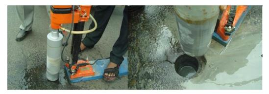
Fig. 5 Core cutting in progress Km 32.350 Chennai-Tada road, N.H.5
