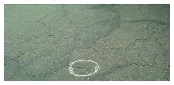
Fig. 2 Alligator map cracking at Km 45.30 Chennai-Tada road, N.H.5
